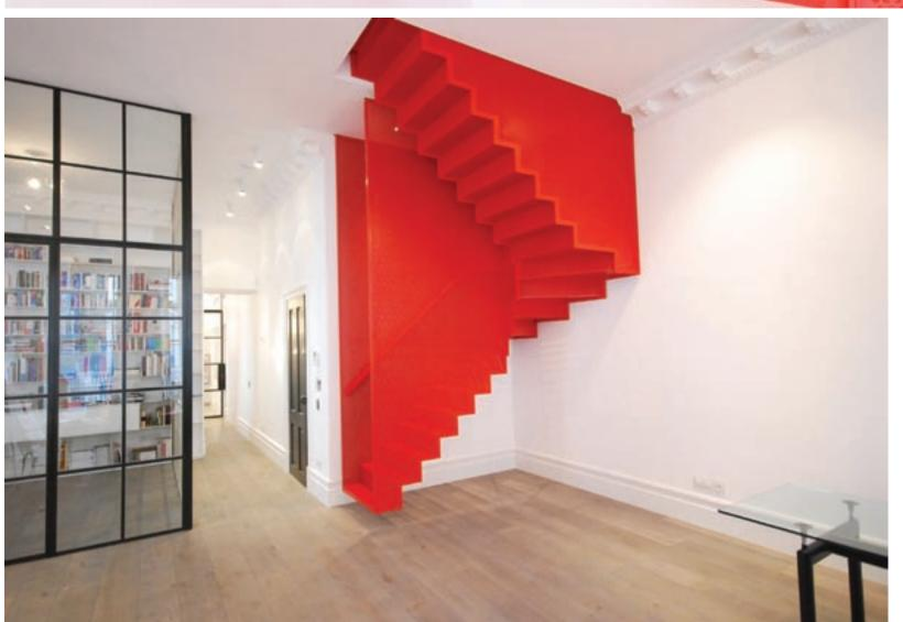
Tasked with creating a staircase for a split level property, our team was set the challenge to produce a staircase completely hanging off the existing building structure.
